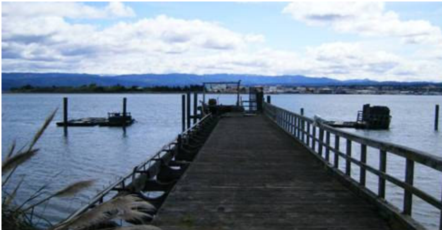
Figure 2-26: Pre-Existing Cogeneration Plant Water Intake Berth
