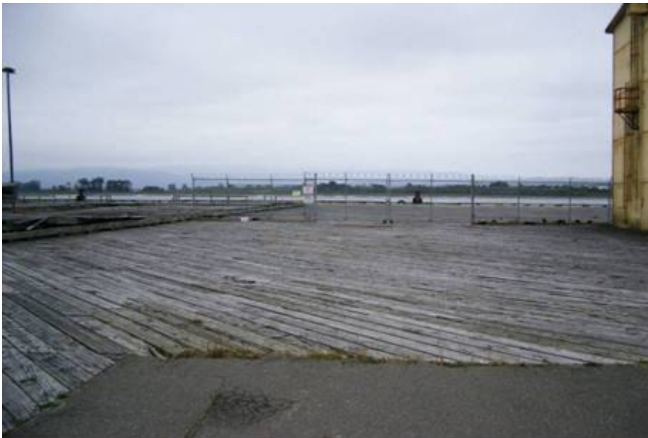
Figure 2-16: Berth 1 Timber Deck
