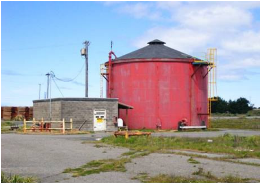
Figure 2-30: Fire Main Pump Station
