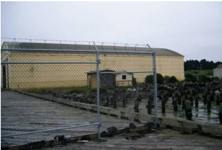
Figure 2-18: Berth 1 Access Control Fencing
