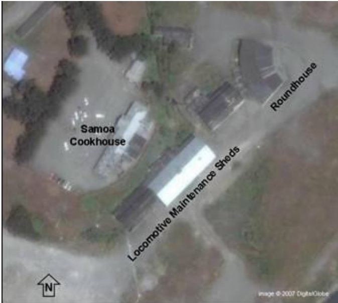
Figure 2-14: Maintenance Sheds and Roundhouse
