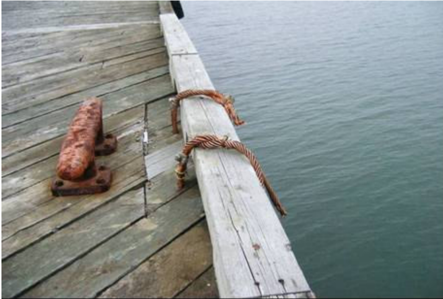
Figure 2-20: Berth 1 Existing Mooring Point
