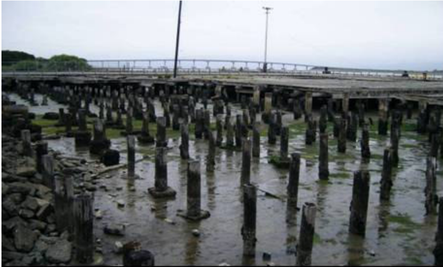
Figure 2-17: Berth 1 Interior Piling Field
