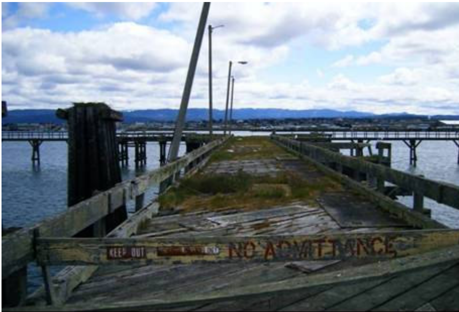
Figure 2-23: Berth 2 Ship Berth Access Pier
