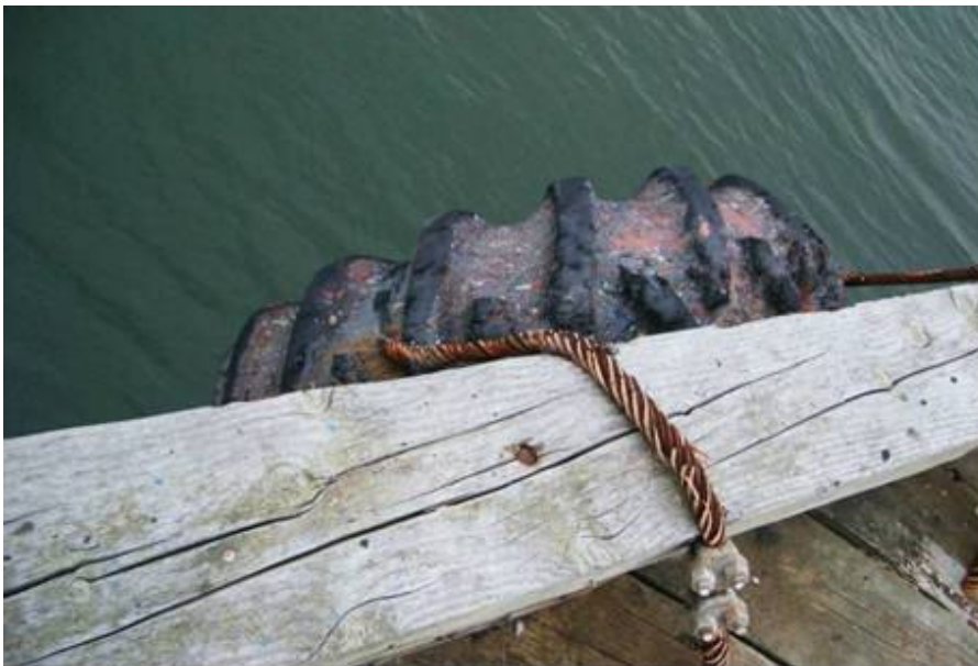
Figure 2-19: Berth 1 Existing Fender System
