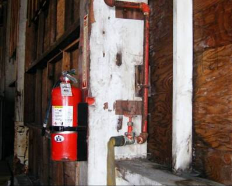
Figure 2-11: Warehouse 3 Timber Columns, Wall Structure and Fire Protection
