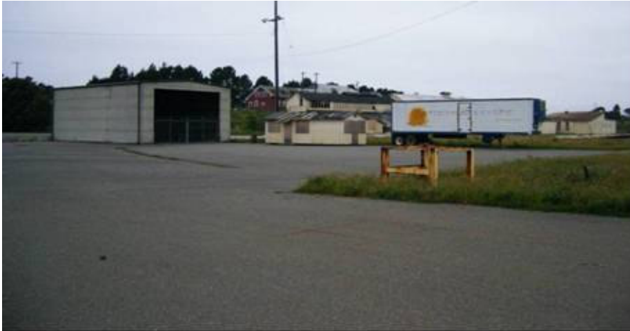
Figure 2-28: Open Storage Pavement North of Warehouse 3
