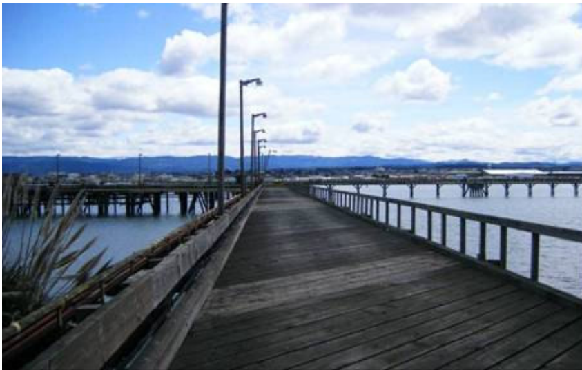
Figure 2-24: Berth 2 – Barge Berth Access Pier
