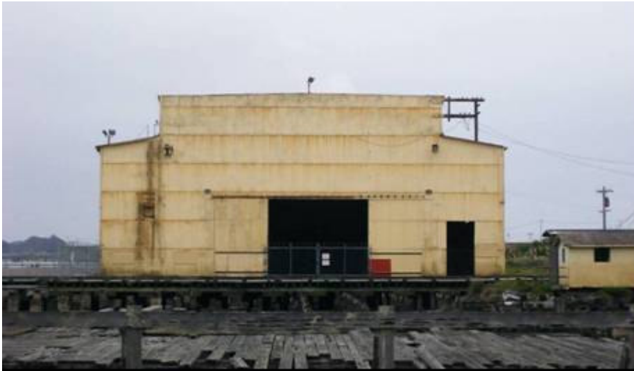
Figure 2-6: Warehouse 14 Existing Pile Supported Pier
