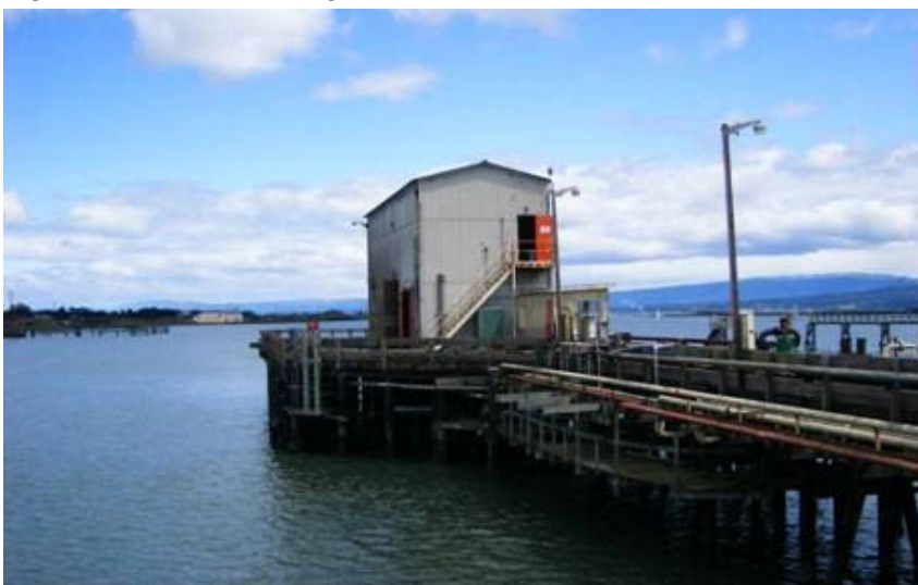
Figure 2-25: Berth 2 – Barge Berth Equipment Shed
